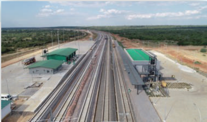
Kipande cha Reli ya Kisasa (SGR) Ruvu Station
